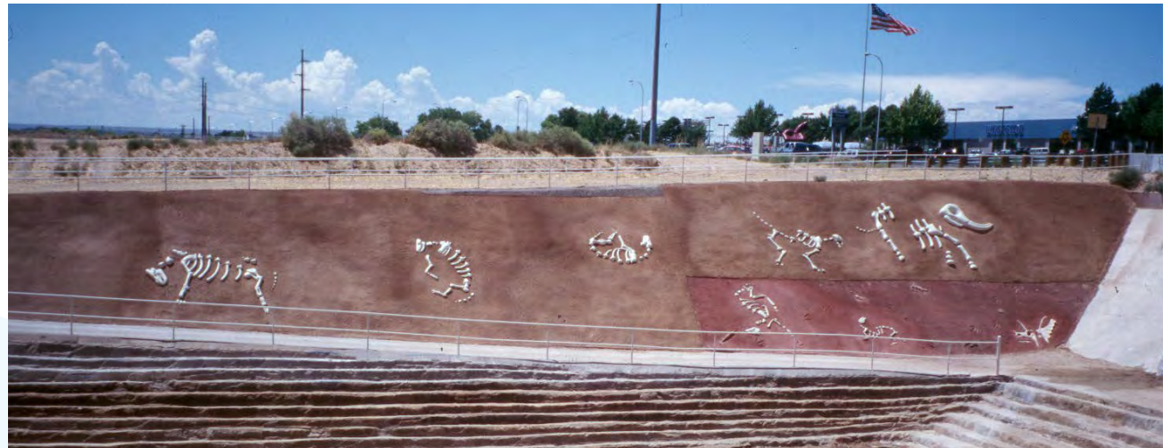
▲ Example of concrete stamping in the river bank to add artistic/creative elements.
