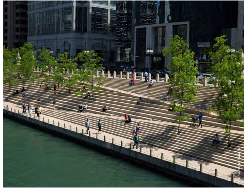
▲ Chicago riverwalk stepped embankment.
