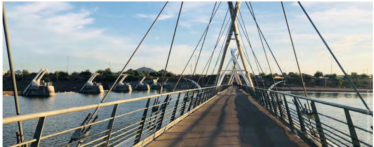
▲ TOP: Option A: Proposed Bike/Pedestrian Bridge BOTTOM: Non-vehicular bridge across Tempe Town Lake.
