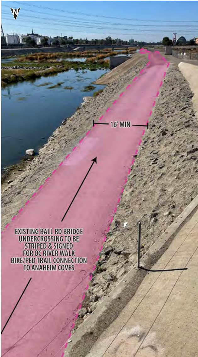
▲ The existing undercrossing at Ball Road bridge to be utilized for trail extension and connection.
