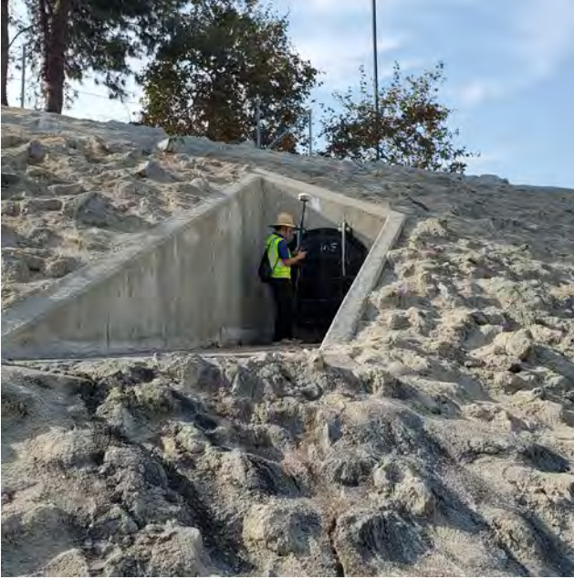
▲ Storm drain invert GPS coordinates were collected for the GIS database.
