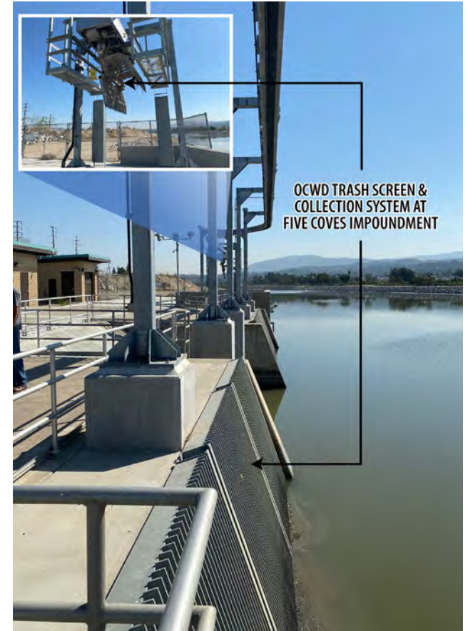
▲ Close up of impoundment O&M at Five Coves location.
