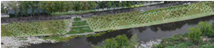
Figure 11: Example of Soil Cement Riverbank Planters that can be Controlled Outside of the River Bottom
