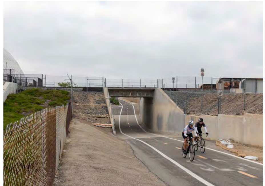
▲ 7B - The existing trail pinch point at ARTIC Railroad crossing.
