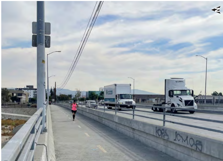
▲ View from west side of Katella Ave. The existing narrow multi-use SART crossing on Katella Avenue.
