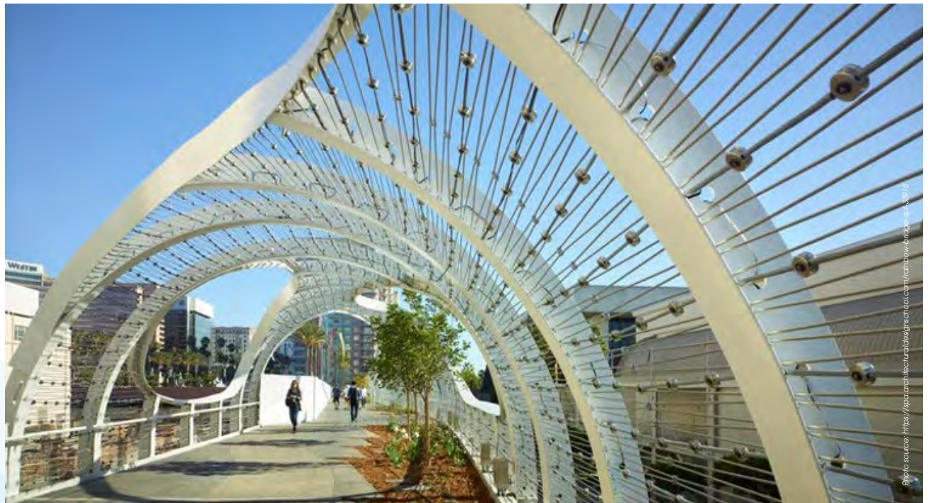
Example bridges, representing the lower and upper cost ranges for a bike and pedestrian bridge.
