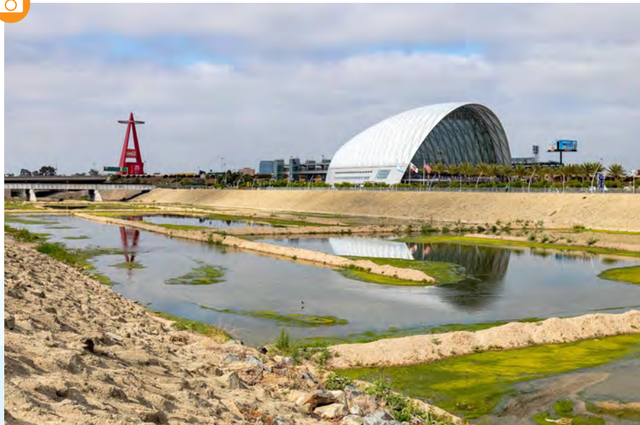
▲ Existing condition Santa Ana River.
