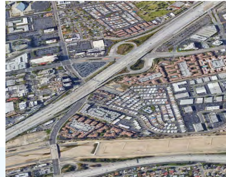
TOP ► Existing Edge Condition along OC River Walk project site.
