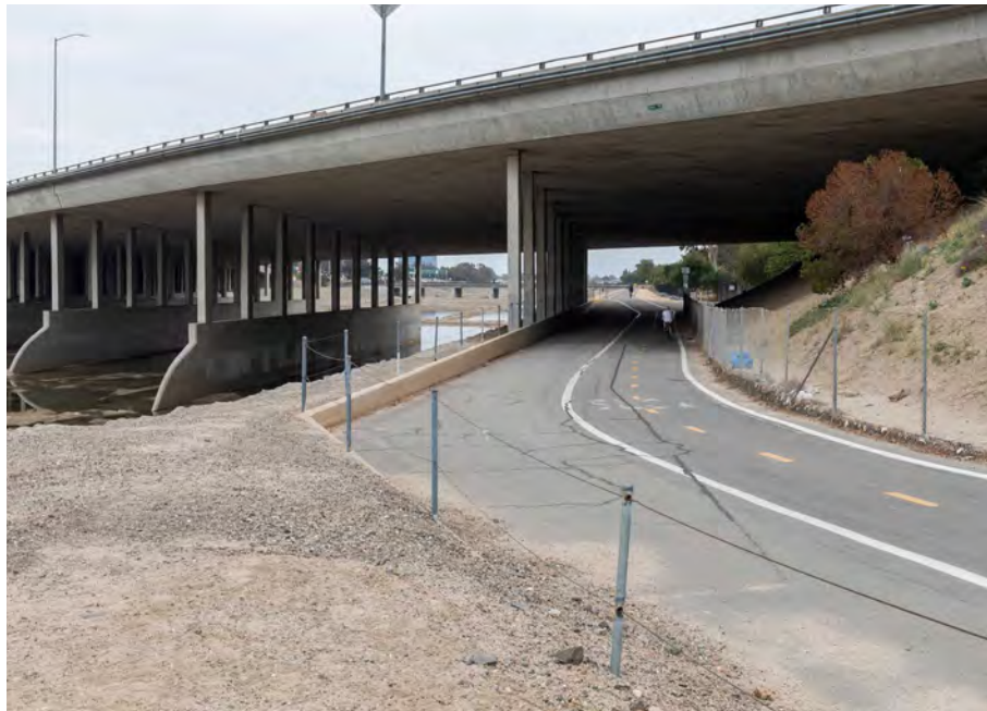
▲ 7A - The existing trail pinch point under the 57 Freeway.
