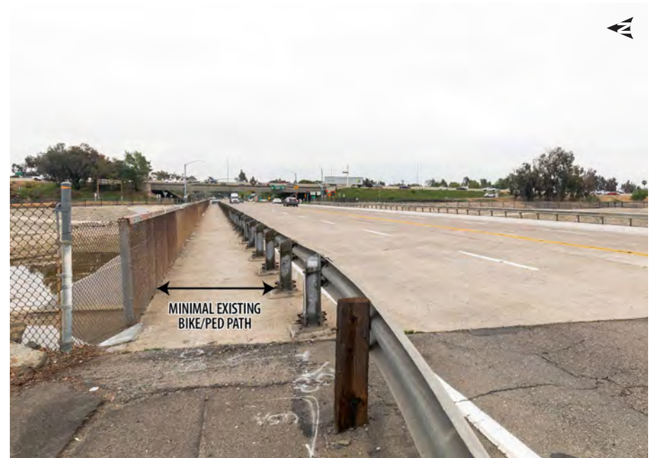
▲ View from Orangewood Ave. bridge at west en. Orangewood Avenue has minimal safety buffer between the pedestrian access and busy traffic.
