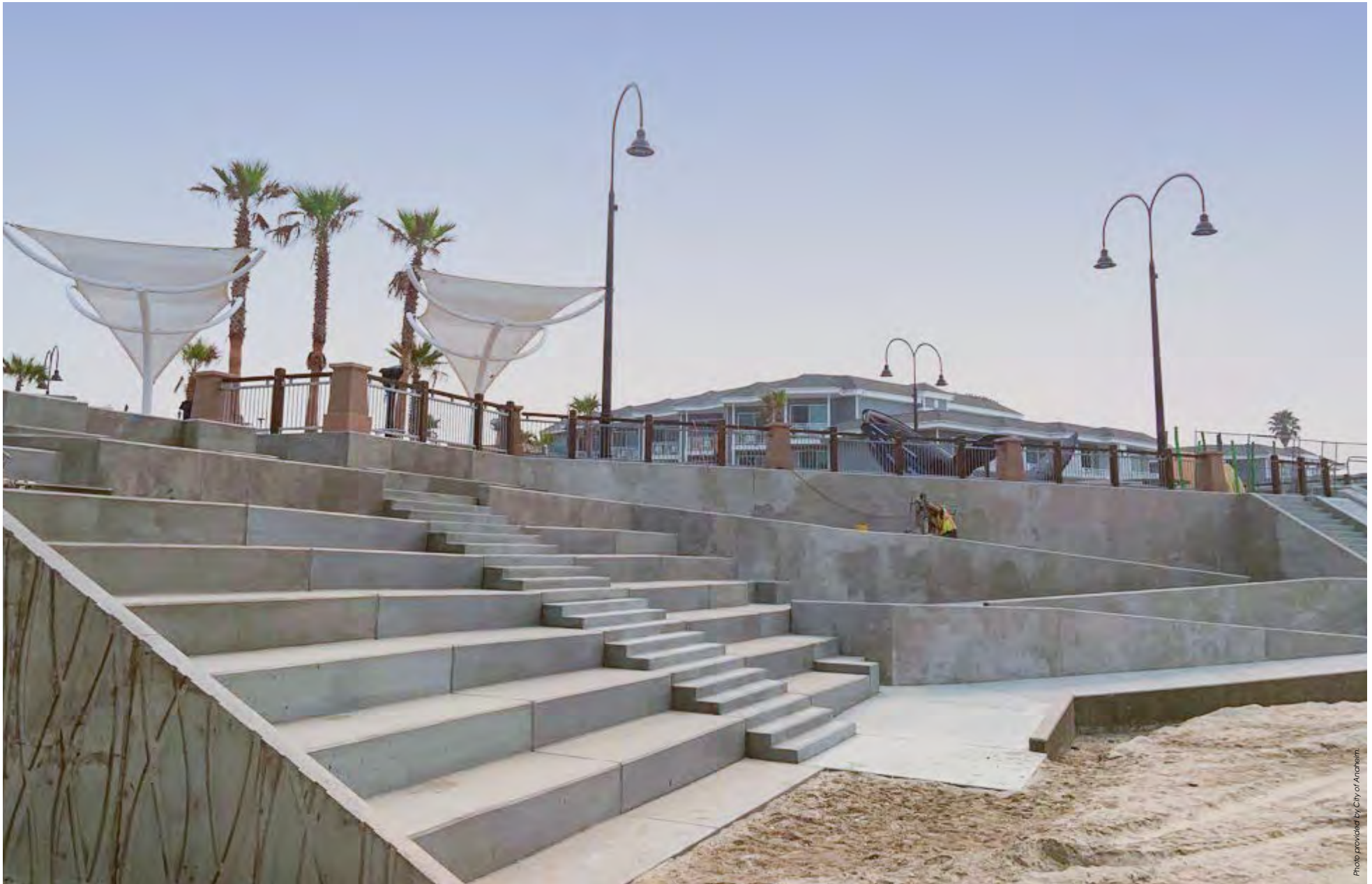
▲ Example of stepped embankment with access to river.
