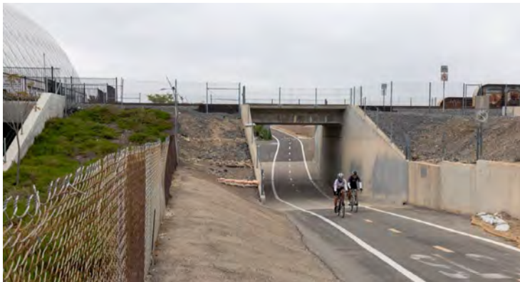
Figure 8: Existing ARTIC undercrossing box – looking North from the SART. The existing undercrossing is narrow and too congested for shared pedestrian and cyclist usage.
