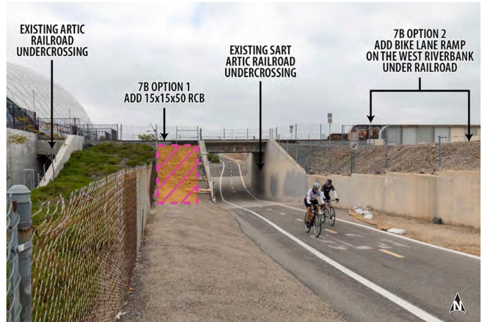
▲ SART from south of ARTIC railroad. The additional box for Option 2 to relieve pinch point congestion can be installed in either of the locations shown.
