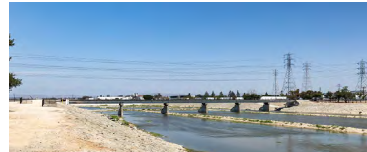
Figure 6: SPT Railroad – looking Northeast from the westerly bank. The eastern undercrossing is visible on the right. The western bank [on the left] does not have an undercrossing, and a black gate/fence prohibits access across the railroad.
