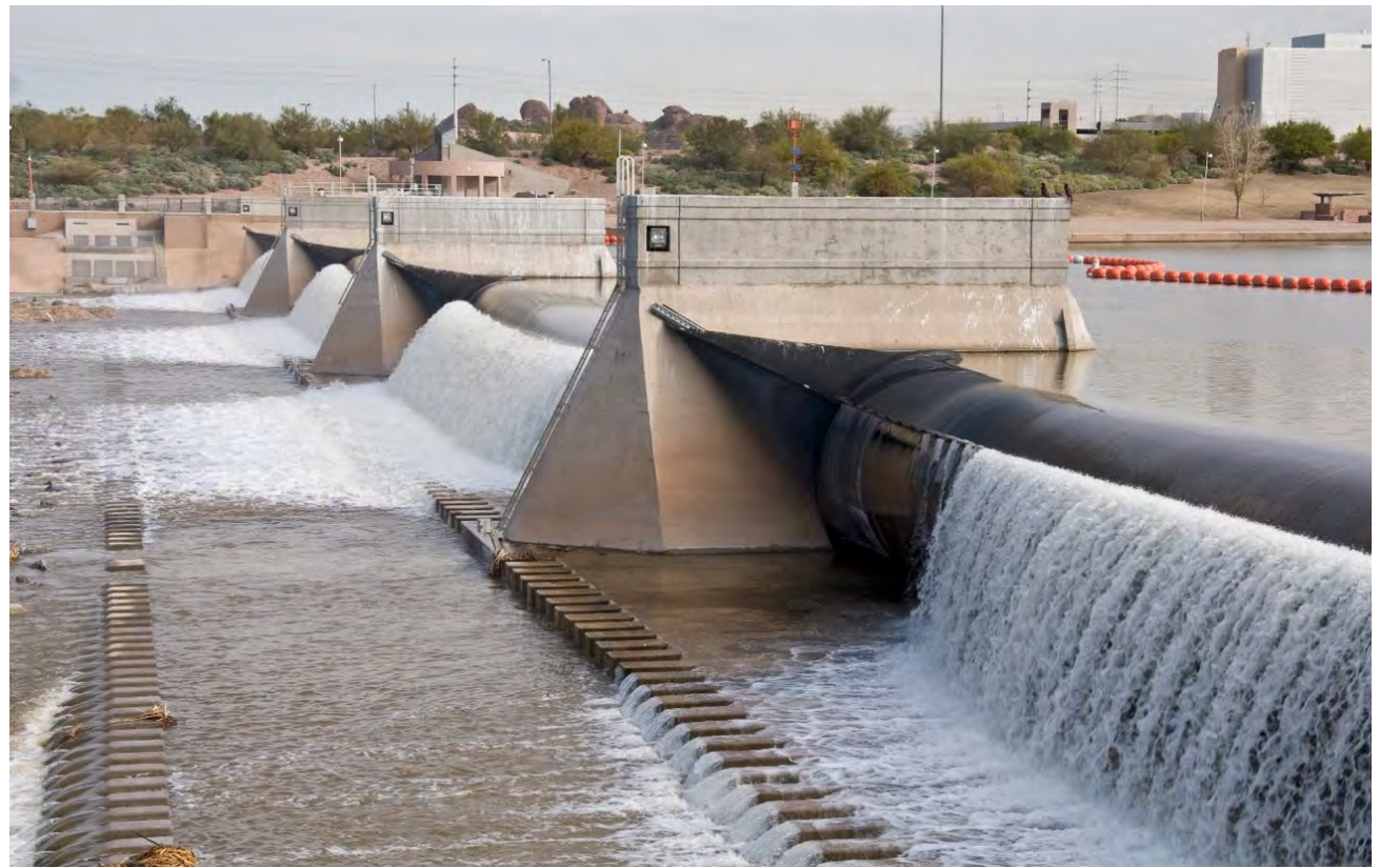
Original rubber dam impoundment system. ▶
