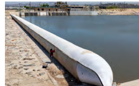
▲ Existing OCWD rubber dam impoundment
