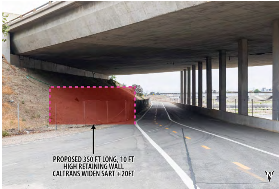
▲ On west bank, looking south at the isometric concept of a retaining wall, to push back the slope and create more trail width.
