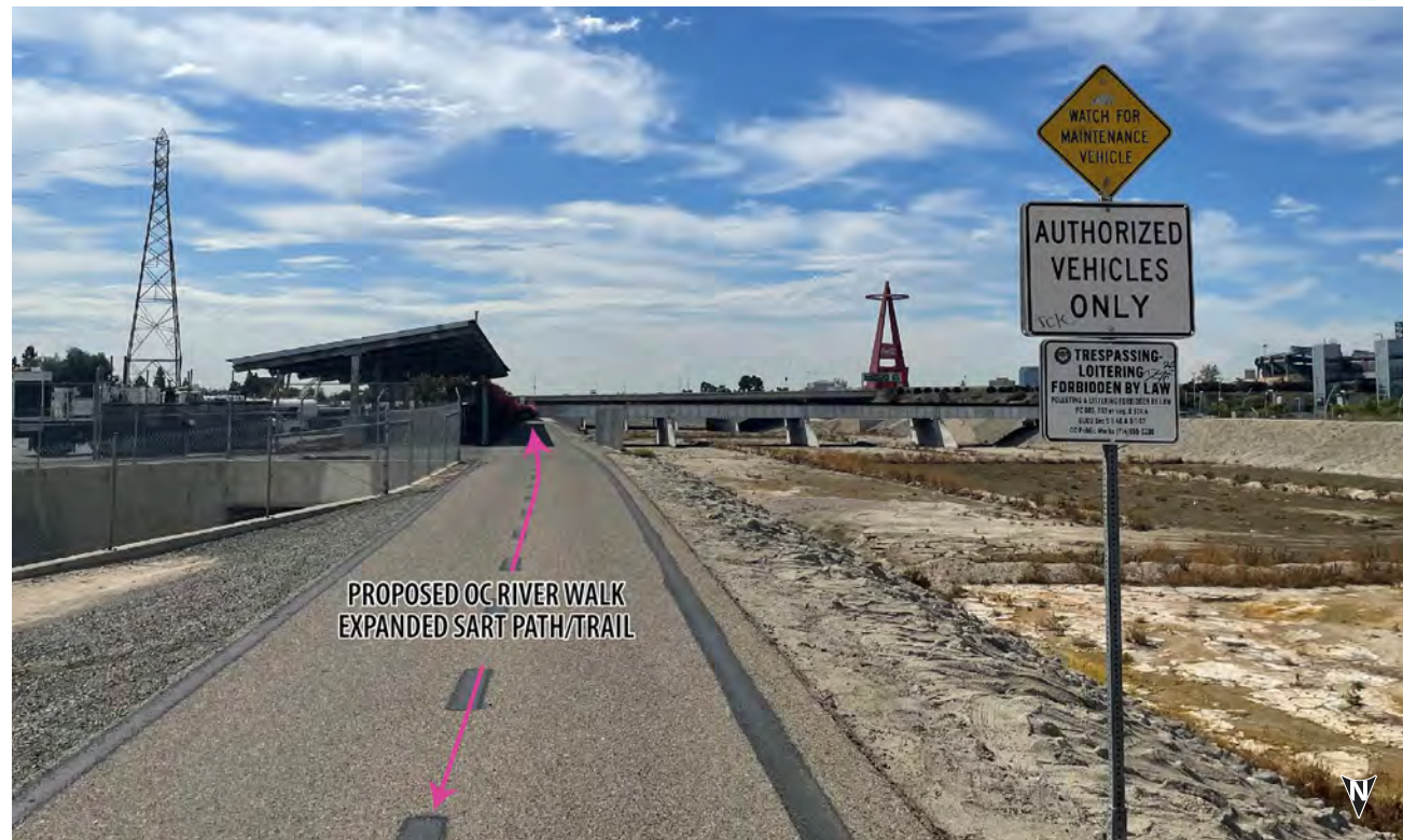
▲ On east bank, looking south at the existing road currently utilized for authorized vehicles only. The footprint width can accommodate OC River Walk trail improvements.
