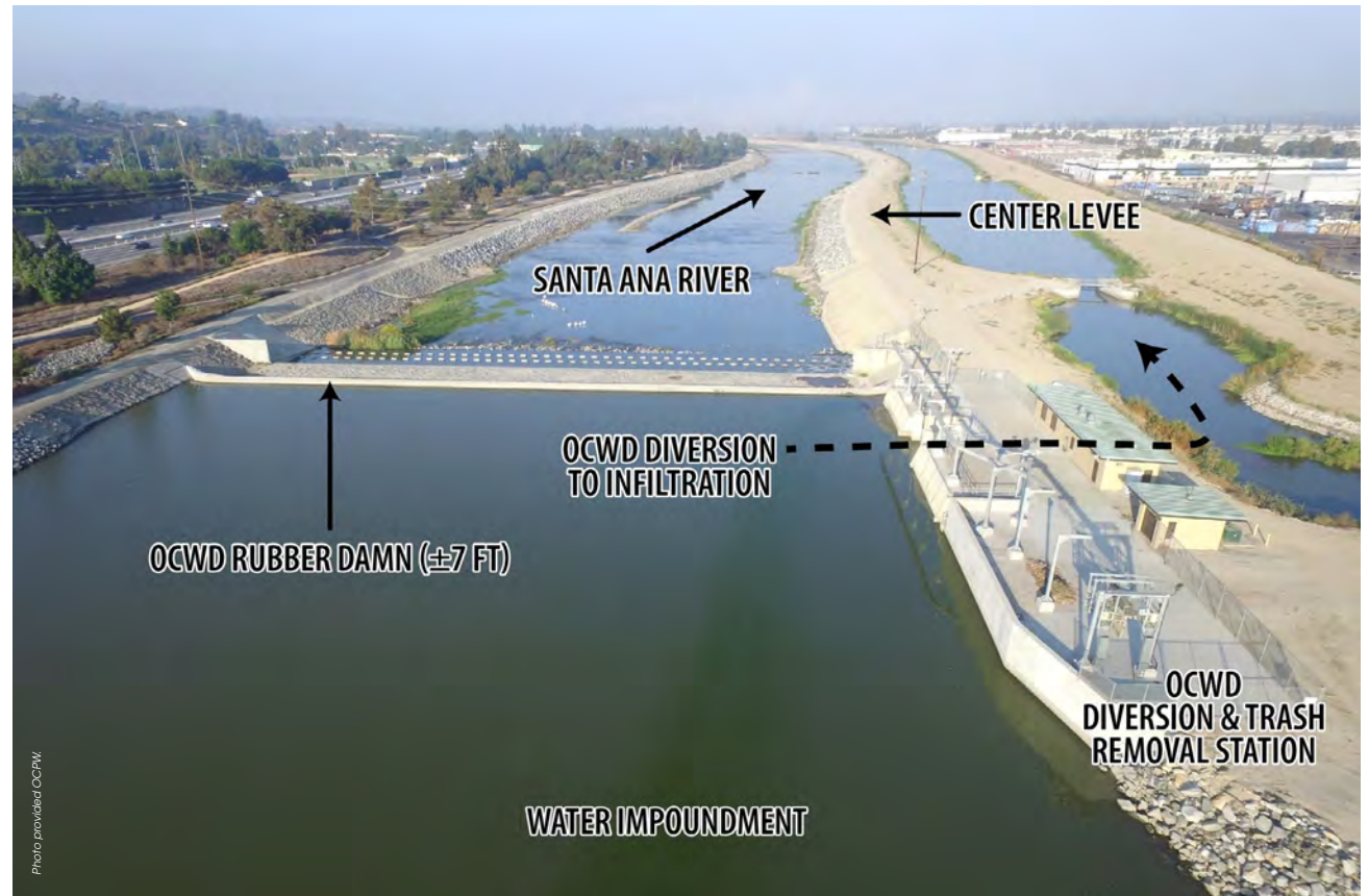
▲ Santa Ana River OCWD rubber dam and impoundment at Imperial diversion.
