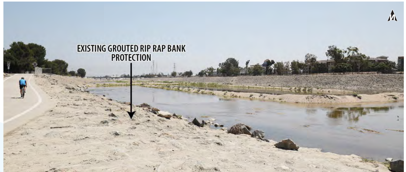
Photo shows the proximity of the existing riprap to the SART
