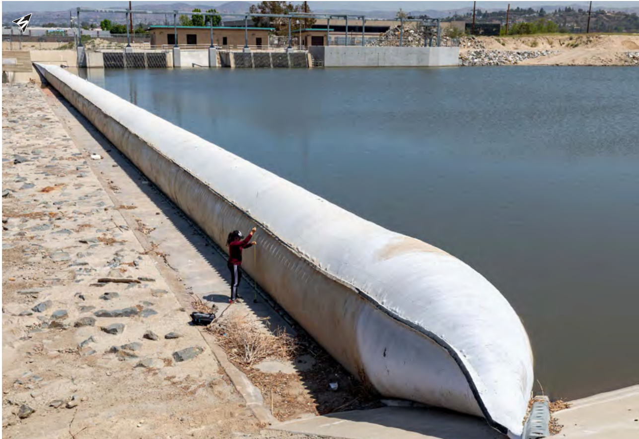
▲ Santa Ana River Imperial Rubber Dam – looking Northeast from the southerly river bank. OCWD operates the seven-foot-high rubber dam and diversion facility for water impoundment and groundwater recharge.
