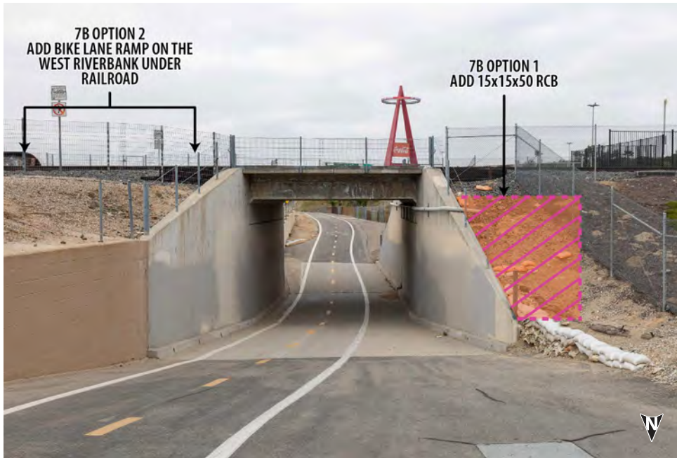
▲ SART from north of ARTIC railroad. The additional box for Option 1 to relieve pinch point congestion can be installed in either of the locations shown.
