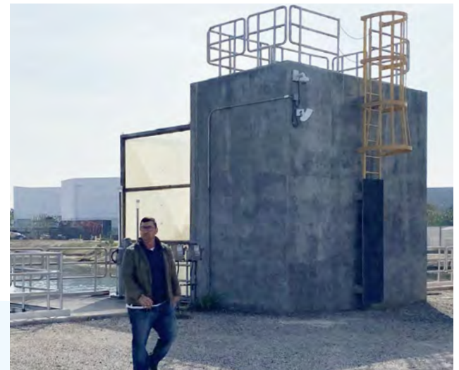
▲ TOP: Ultra clear and clean GWRS water. BOTTOM: OCWD-GWRS turn out structure.
