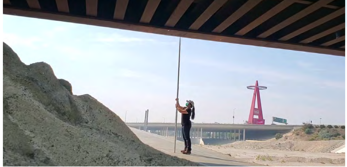
▲ Bridge undercrossing measurements were taken to establish available freeboard and minimum height requirements for maintenance vehicles.
