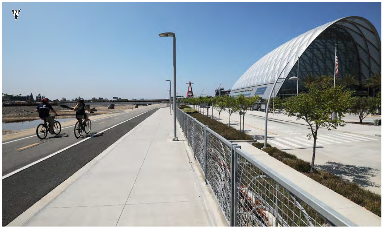
▲ View from west bank of river near ARTIC parking lot on SART. Currently, commuter cyclists already utilize the full width of existing striped trail. The existing space on either side of the trail is not designated or utilized.
