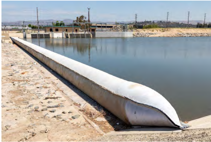
Figure 2: Santa Ana River Imperial Rubber Dam – looking Northeast from the southerly river bank. OCWD operates the seven-foot-high rubber dam and diversion facility for water impoundment and groundwater recharge.
